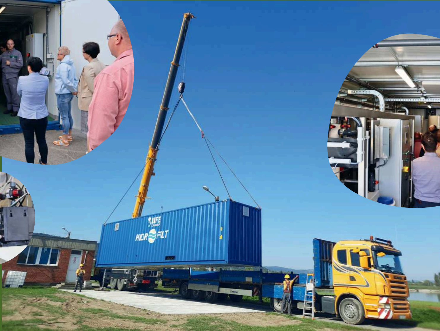
Prototype II. installation site
